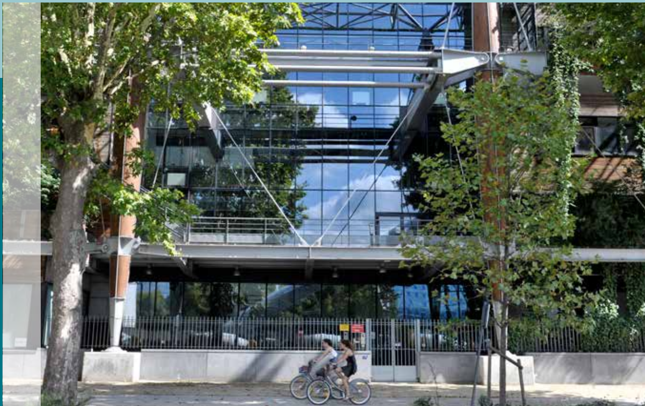
Isséane waste recovery centre in Issy-les-Moulineaux.
