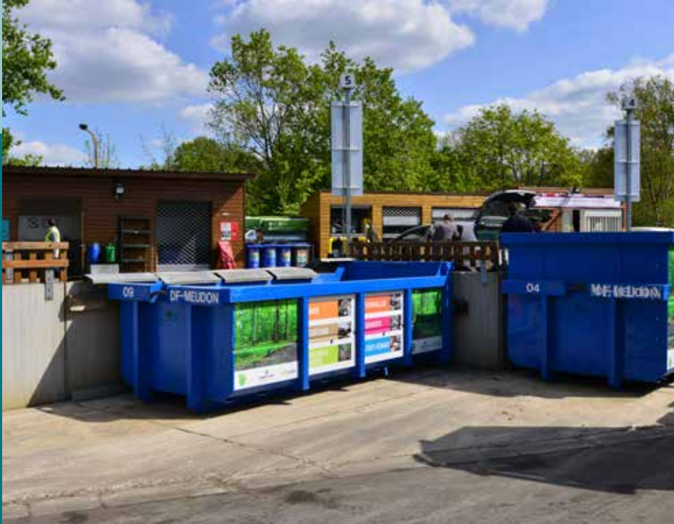
The Meudon waste reception centre, transferred by Syelom to Sycotom on 1 January 2017
