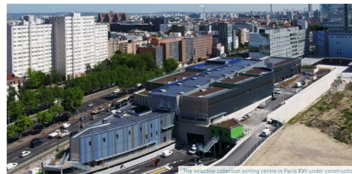
The selective collection sorting centre in Paris XVII under construction
